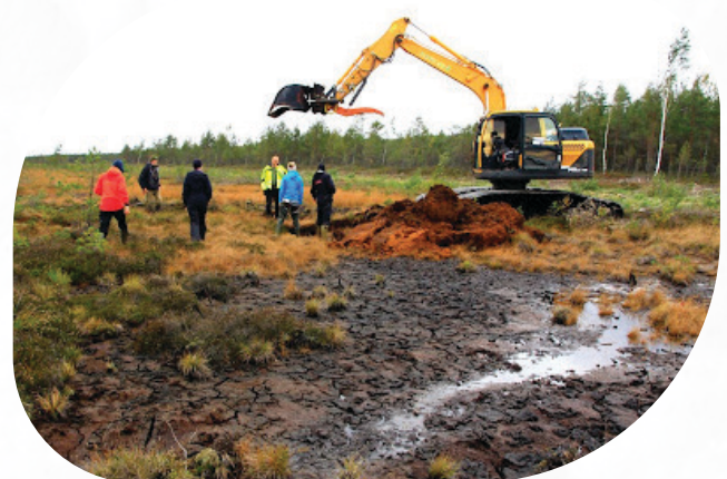
Ditch damming works in the northern part of Soosaare bog in 2018, on a former cut-over peatland. Taken by: Edgar Karofeld (University of Tartu)
